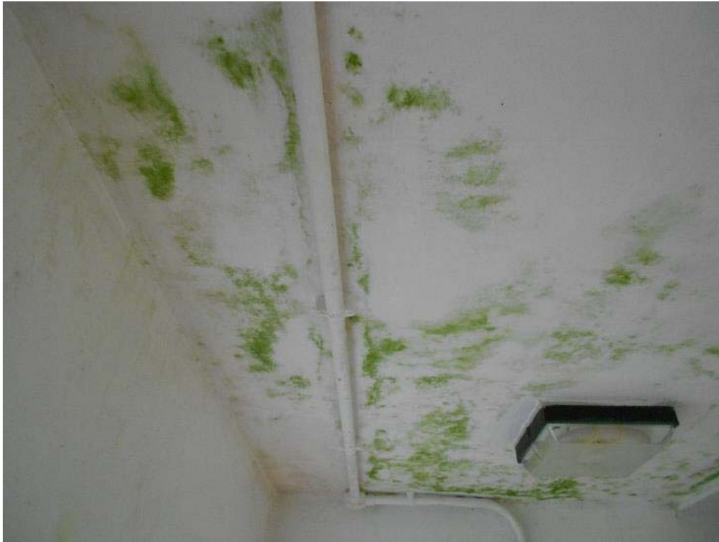
Ceiling in A wing shower room
